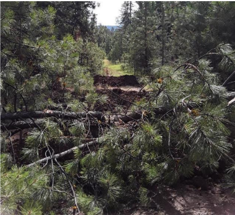
Figures 27 and 28: Multiple tactics were utilized to reduce and prevent unauthorized motor vehicle use of closed roads within the project area. Pictured here are examples of multiple berms, and the placement of slash, debris, and boulders to secure the physical closures. In addition, two gates were placed on the landscape to allow for continued, but infrequent, administrative access when needed.
