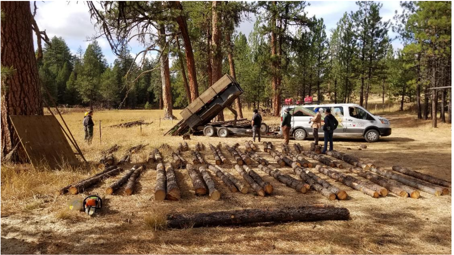
Figures 9, 10, and 11: Members of the Heart of Oregon – AmeriCorps group assisted the U.S. Forest Service in construction of a half-acre buck and pole fence that excluded wildlife from a portion of the meadow that had some existing hardwoods which were heavily browsed as well as newly transplanted aspen and other hardwoods as part of the restoration efforts. Materials were sourced from onsite, using conifers encroaching into the meadow as the fence poles and rails.
