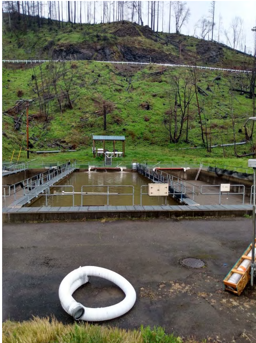
Figure 2.3. Picture of intact raceways and ultraviolet (UV) ozone system in front of Rock Creek Road, April 2022. The small ozone structure with the green roof is the same one shown in the above pictures from the FEMA report, with burned trees removed and the road more visible, along with visible debris slides at the road level.
