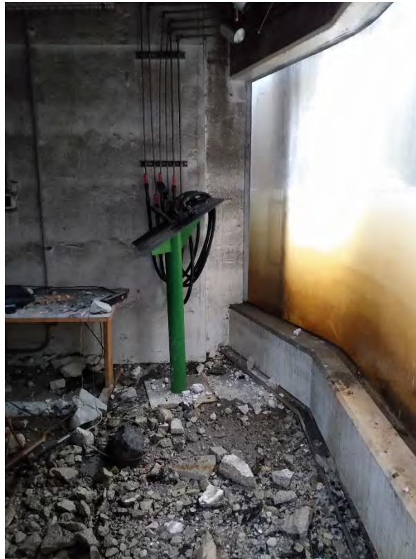
Figure 1.10. Viewing window by dam and fish passage with burned wiring and computer and video equipment used in fish counting.
