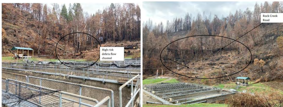
Figure 2.2. Photos of Rock Creek Hatchery showing potential debris flow and landslide areas considered a high risk due to destabilized soils and erosion potential (FEMA 2020).
